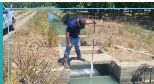
Matt Dermody takes a reading with a staff gauge at the weir where a grower is taking water. The difference between measurements taken above and below the weir reveals how much water is used.
