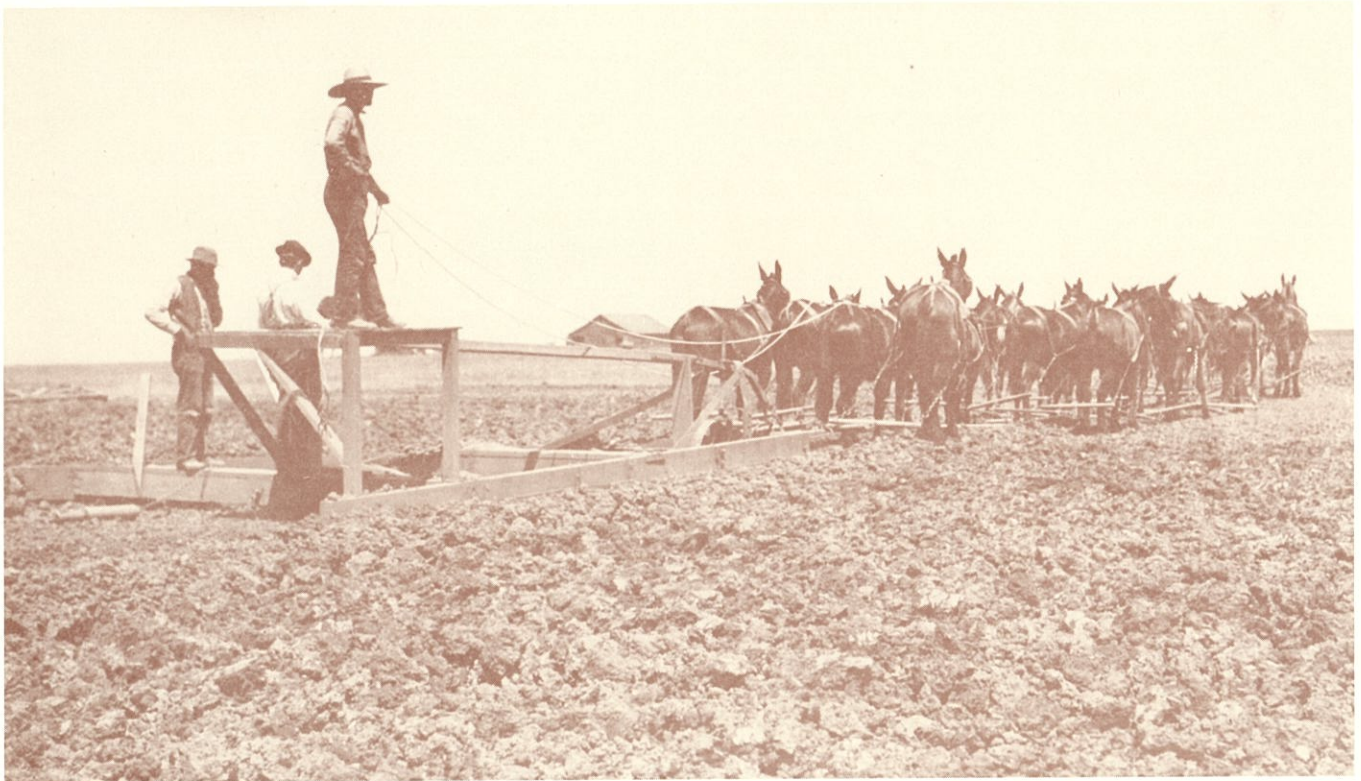
Mule-drawn land plane preparing for irrigation
