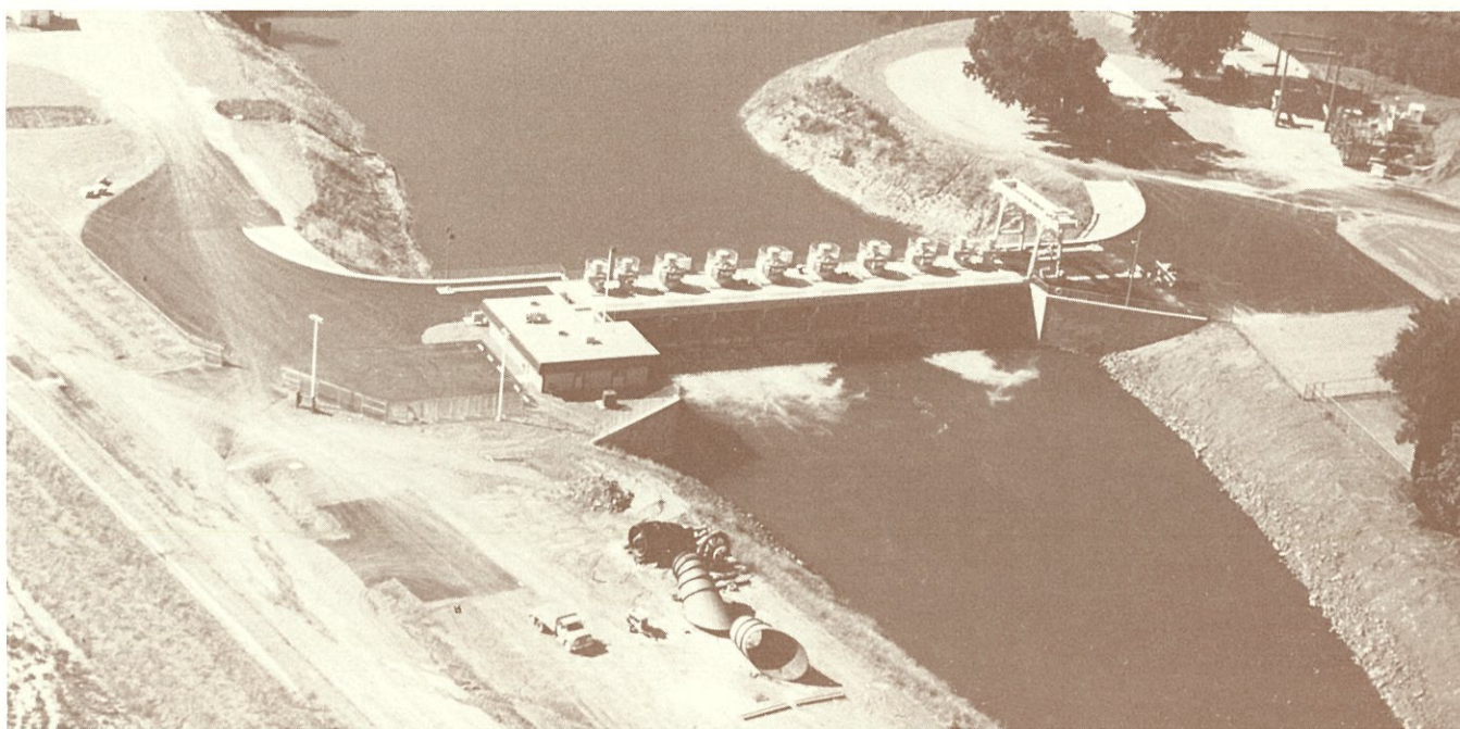
A view of the completed pumping plant; old pump No. 7 is being assembled for historical display in foreground. (Courtesy of R.G. Fisher Construction Company)
