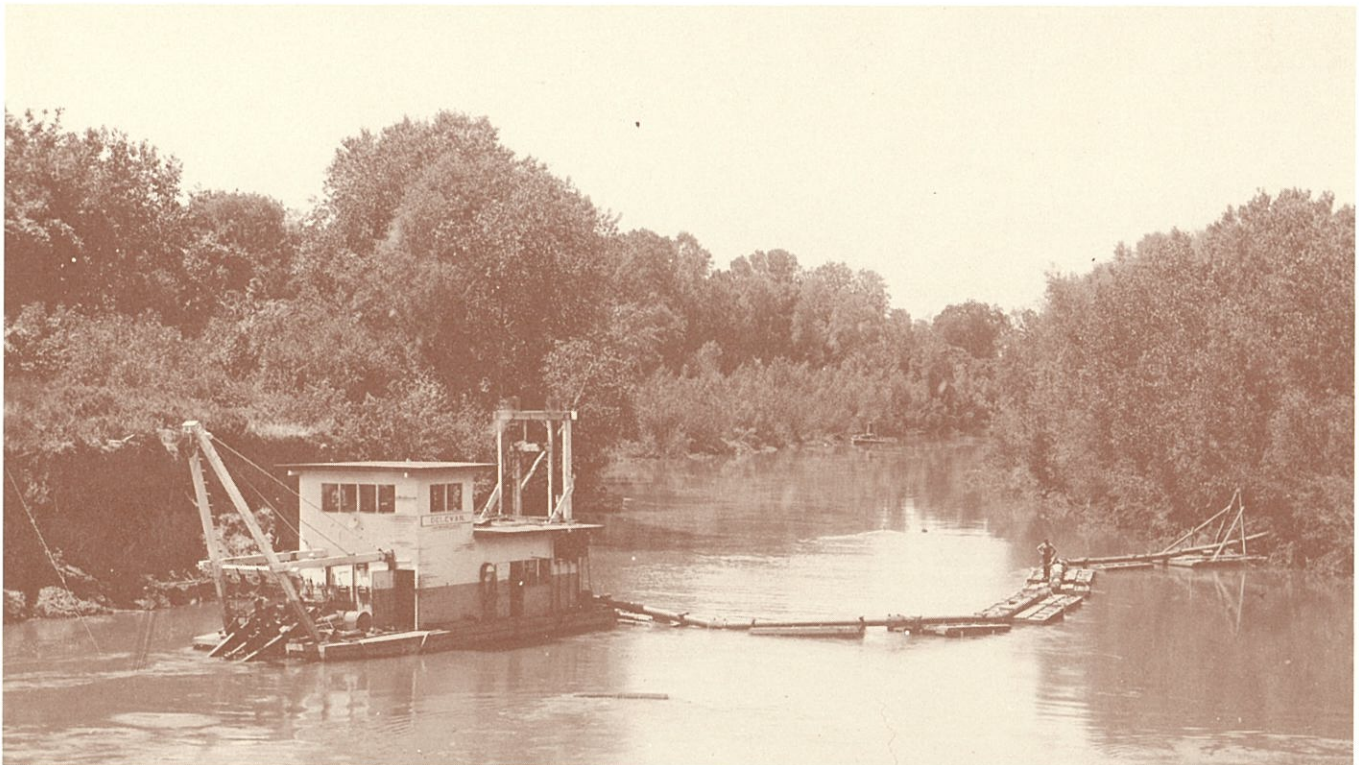
The Dredge "Delevan" cleaning Intake Channel, on June 27, 1918
