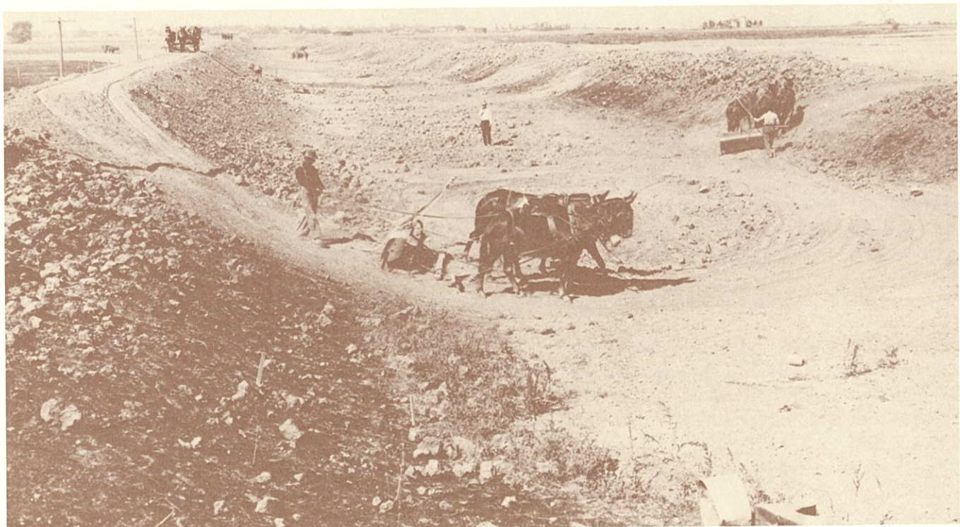
The main canal being excavated with fresno scrapers
