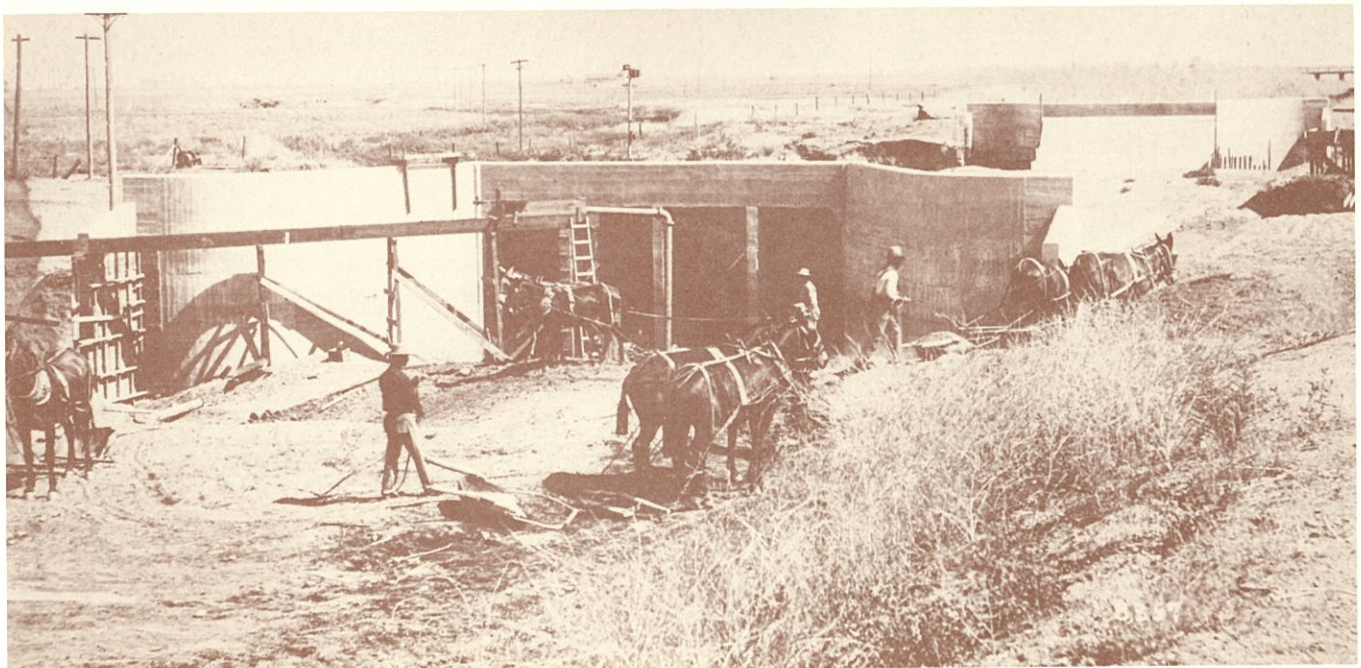
Siphon nearing completion
