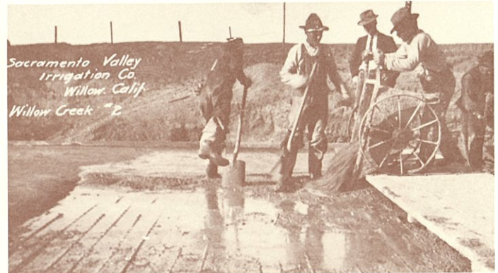
Placing concrete to finish top of Willow Creek Siphon
