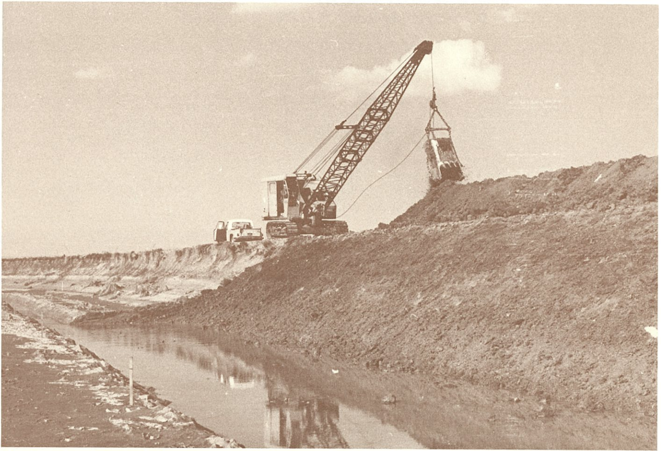
Dragline at work on canal enlargement and rehabilitation
