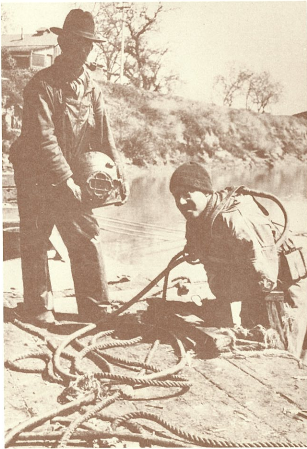
Diver inspecting channel for snags, from Dredge "Delevan"
