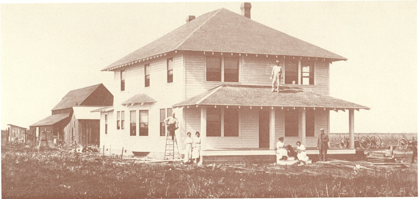
The Otterson family at work as house nears completion
