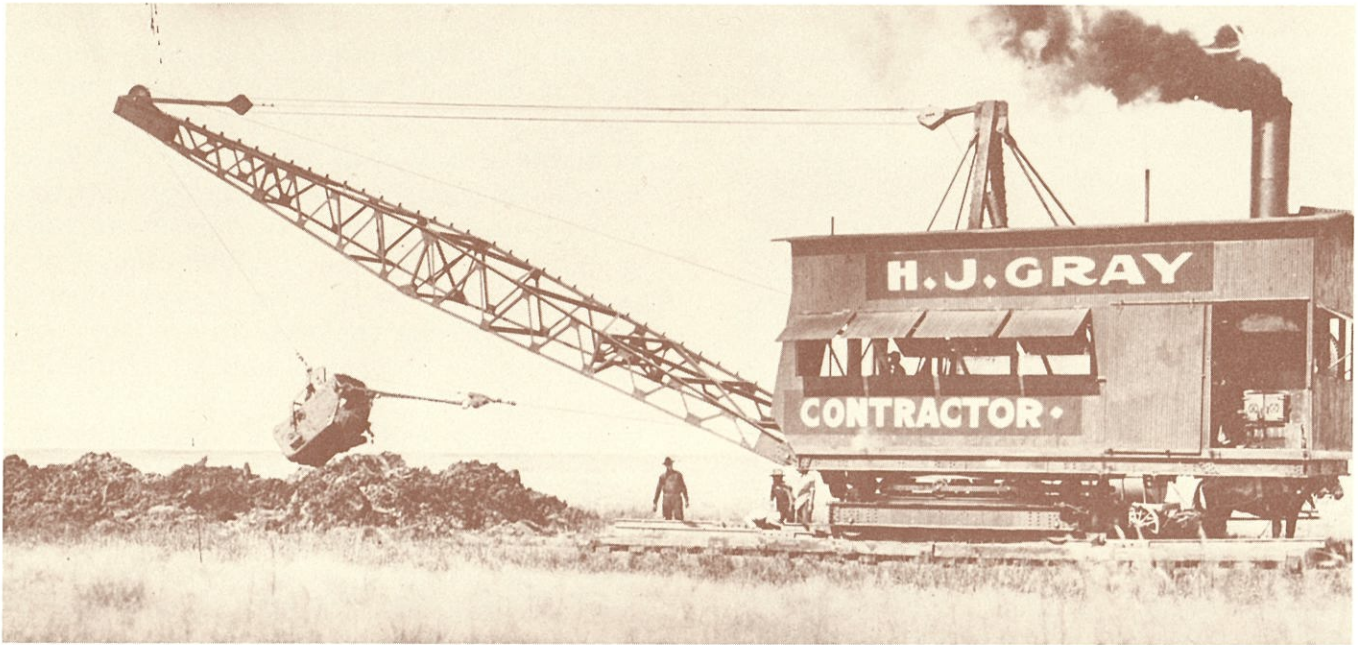
Steam dragline excavating canal
