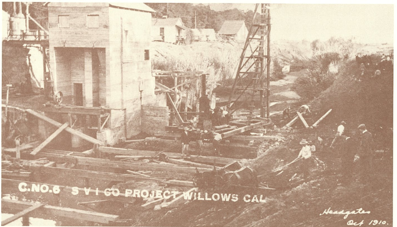
Construction of pumping plant at headgates, October 1910
