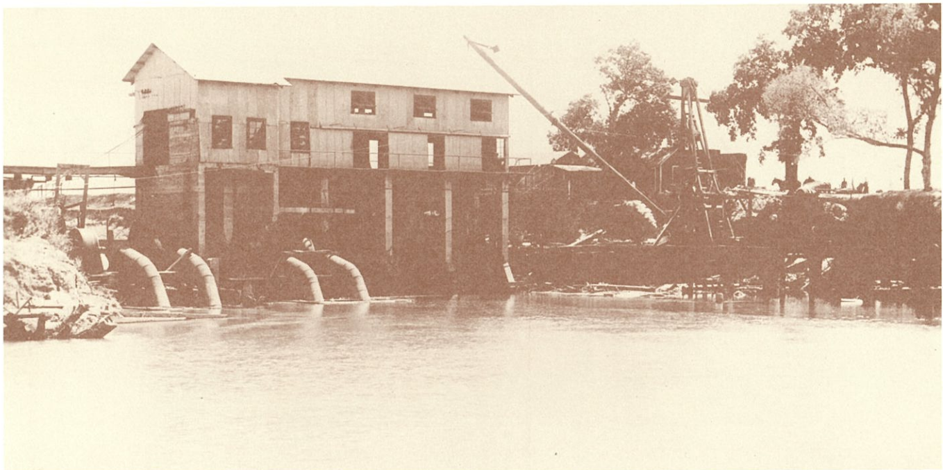
View of pumping plant, derrick and steam pile driver, June 13, 1919
