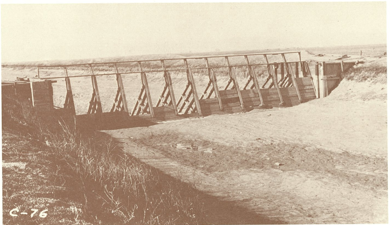
Timber check structure, January 18, 1920
