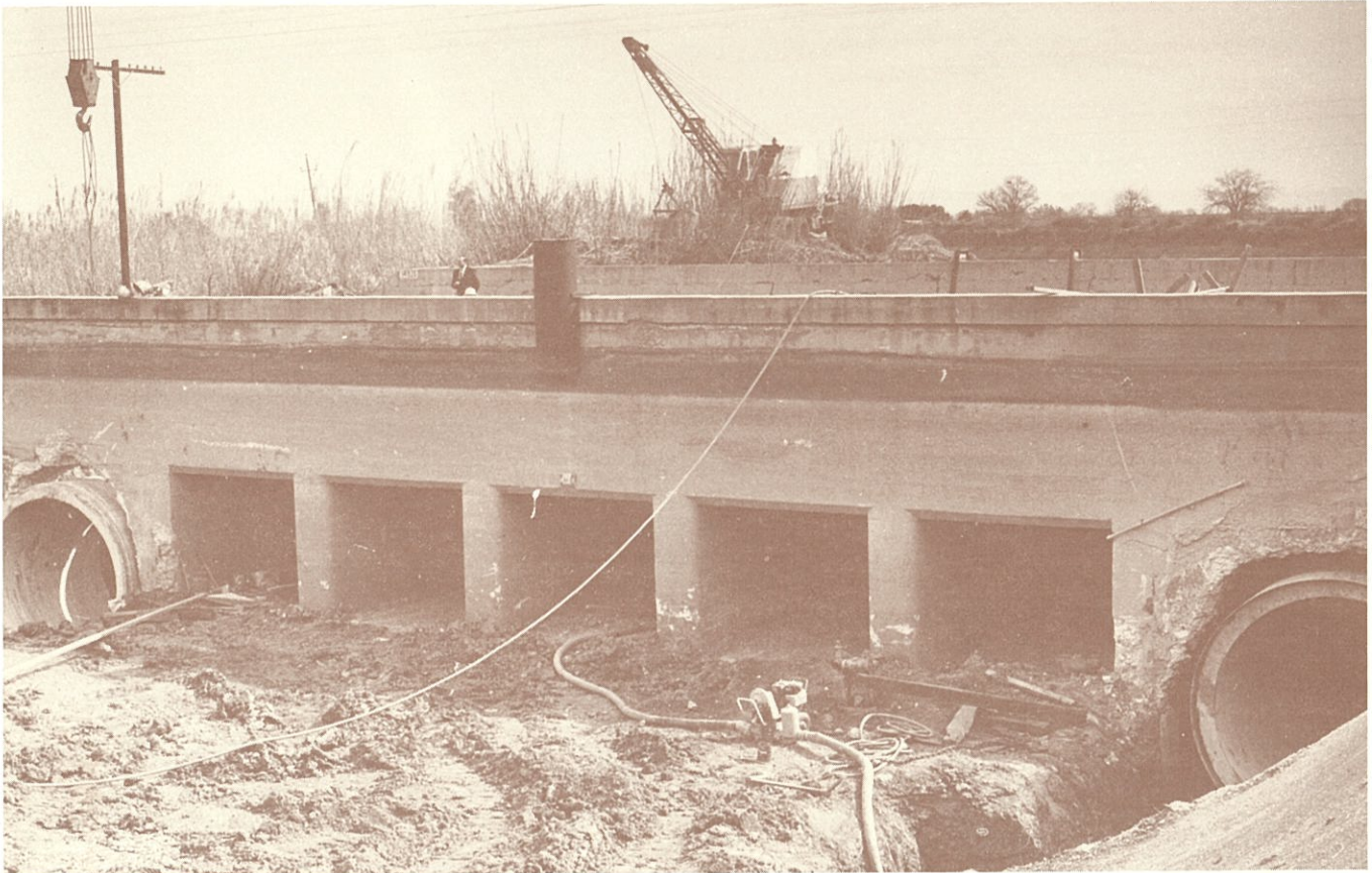
Enlargement of railroad siphon, 1967-68
