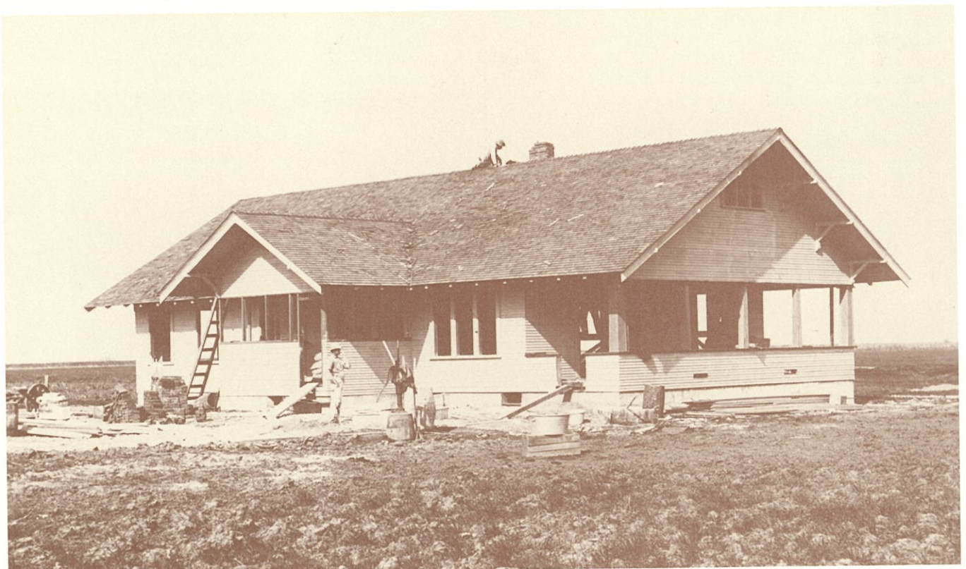
The Pelko residence under construction
