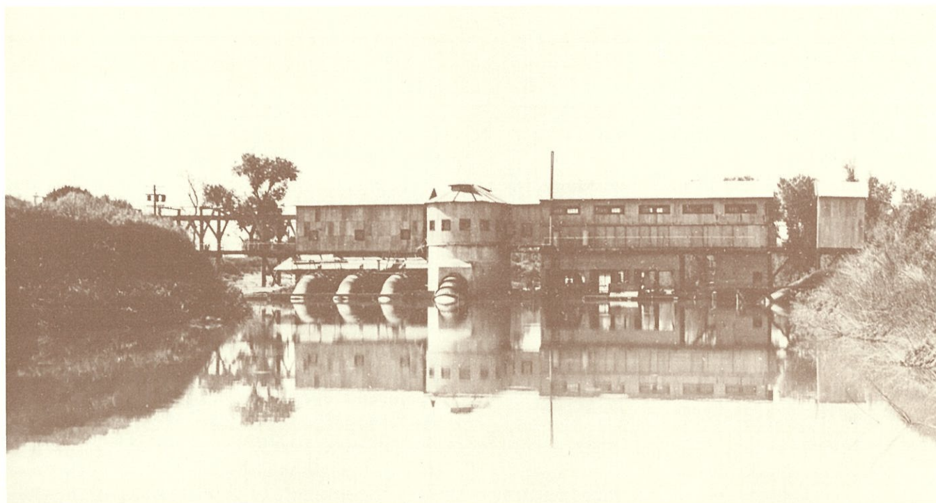
Downstream (discharge) side of main pumping plant in early 1930's
