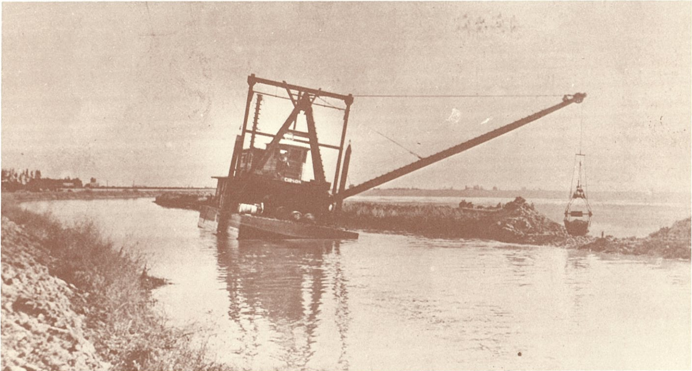
Dredge "Gibson" closing gap in canal (named after Director Gion Gibson)
