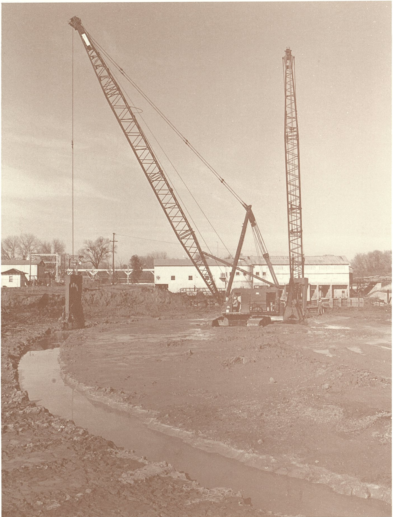
One hundred foot deep slurry trench in progress, January 8, 1982
