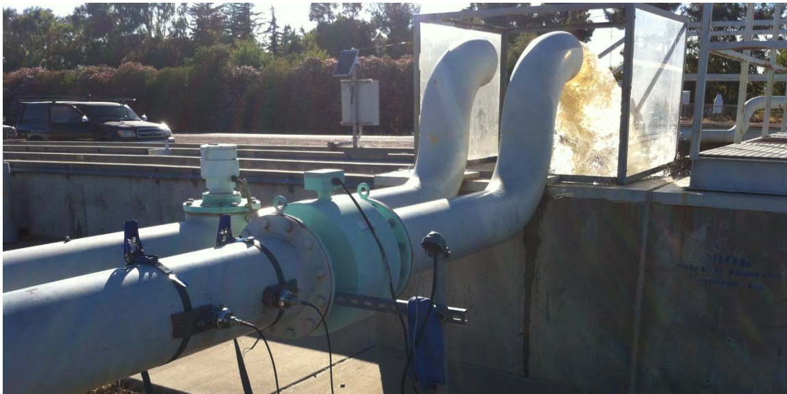
Figure A-4. Water Specialties Magnetic Flow Meter at CSUC ATRC
