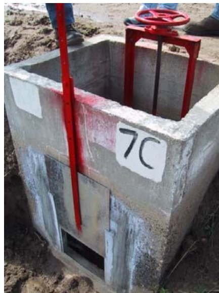
Figure 28. Alta ID rectangular orifice gate (front) provides flow measurement, while sluice gate (rear) provides flow control
