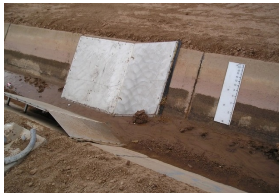
Figure 46. Flat-bottomed (actually, a “Vee” in this case) flume immediately after construction. The sediment will flush out once water flows in the ditch.
