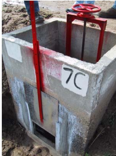
Figure 16. CHO at Alta ID. The orifice (on the canal, upstream side) is a standardized rectangle with an adjustable, bolt-secured opening. The downstream gate with the round handle is used to adjust the flow rate to the target.
