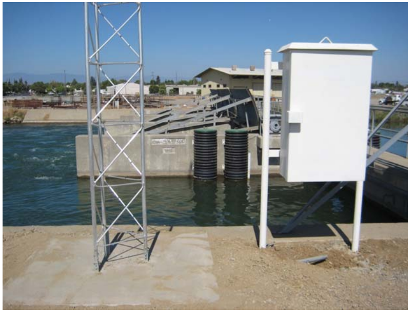
Figure 3. Automated radial gates on Glenn Colusa ID main canal at IID. Radio tower and instrumental enclosure for a PLC are in the forefront.
