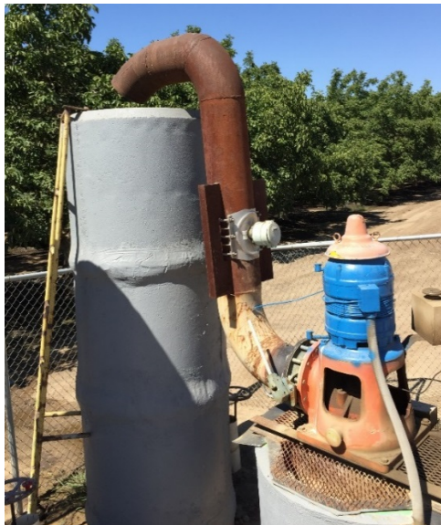
Figure 4. Propeller meter with a vertical orientation
