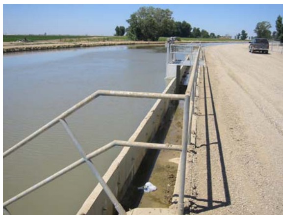
Figure 6. Special entrance to a 200 AF regulating reservoir at Central California ID. The sluice gates in the center are automated to open if the water level gets too high. Pumps at the upper right hand side (not seen) empty the reservoir if the water level in the canal gets too low. The long walls are for emergency spill into the reservoir.
