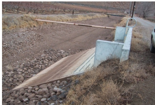
Figure 9. Punch plate at the inlet to an irrigation district lateral pipeline. 1 inch holes, 50% open area, to maintain less than 0.5 ft/sec through the holes (0.25 ft/sec approach velocity).
