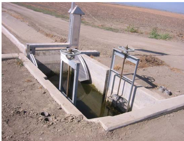
Figure 2. Example of an automated flow control turnout, with two adjacent manual turnouts
