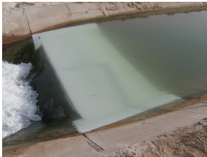
Figure 40. A flume with an ePaint™ coating to minimize algae growth
