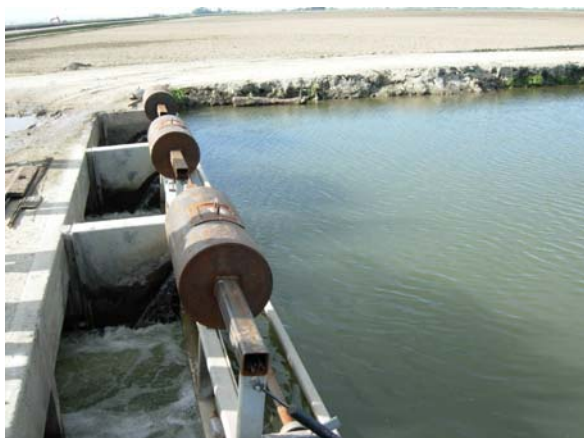
Figure 5. Three ITRC flap gates in parallel at San Luis Canal Company. These require no electricity, but must have a drop. There are hundreds of these throughout California.
