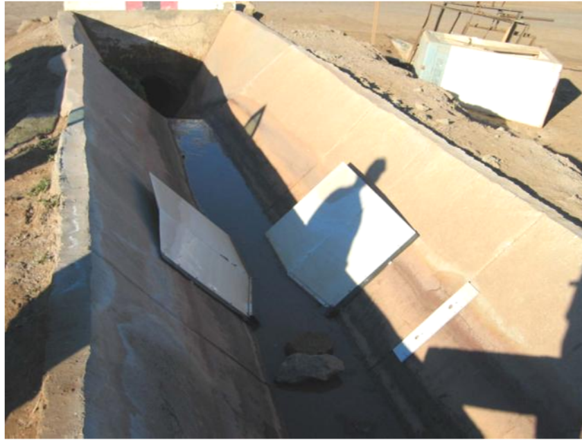
Figure 3. Side contractions rather than a traditional "Replogle Flume". Designed by USBR, Yuma. The rocks are not part of the design.
