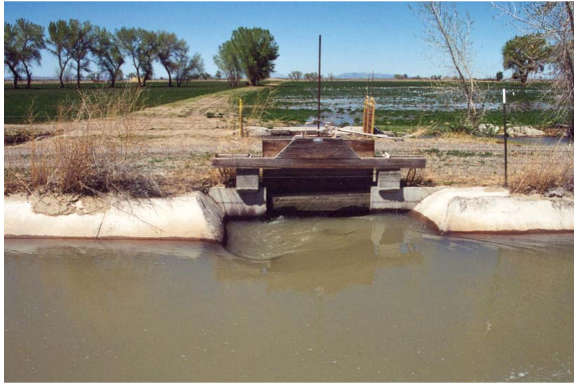
Figure 7. Example of poor entrance conditions into a field turnout. This is not in California.
