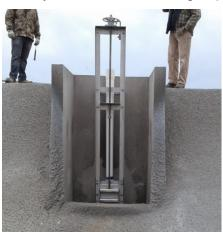
Figure 24. Installed pre-fabricated canal metergate (Fresno ID, 2019)
