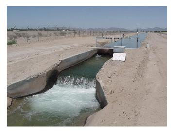
Figure 43. Example of a suppressed weir. The upstream channel has the same width as the weir crest. In this particular case, the walls diverge immediately downstream of the weir, so the nappe is aerated.
