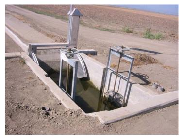
Figure 2. Example of an automated flow control turnout, with two adjacent manual turnouts
