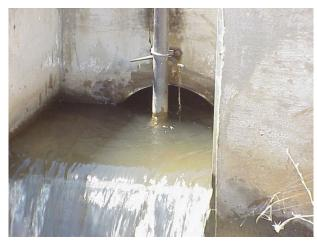
Figure 7. Weir boards are installed downstream of an open propeller meter. Obviously, these are not high enough to create a full pipe condition.
