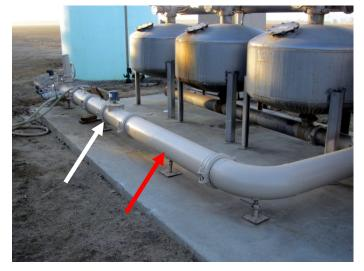
Figure 3. A propeller meter (white arrow) installed downstream of drip system filters, with a long, straight pipe section upstream of the meter (red arrow)
