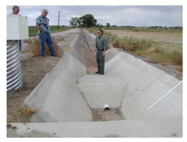
Figure 38. A "Replogle flume" installed on a ditch with high flows in Truckee-Carson ID in Nevada. This is constructed in a trapezoidal section of canal.
