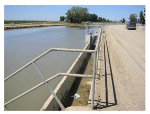
Figure 6. Special entrance to a 200 AF regulating reservoir at Central California ID. The sluice gates in the center are automated to open if the water level gets too high. Pumps at the upper right hand side (not seen) empty the reservoir if the water level in the canal gets too low. The long walls are for emergency spill into the reservoir.
