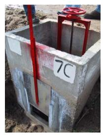
Figure 16. CHO at Alta ID. The orifice (on the canal, upstream side) is a standardized rectangle with an adjustable, bolt-secured opening. The downstream gate with the round handle is used to adjust the flow rate to the target.
