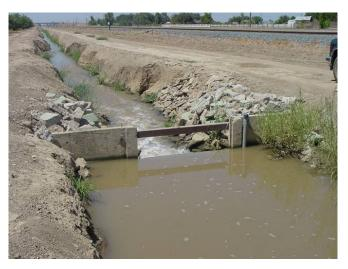
Figure 44. Example of a rectangular contracted weir
