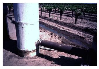
Figure 47. The discharge pressure of the pump will change over time with this type of direct connection to a standpipe
