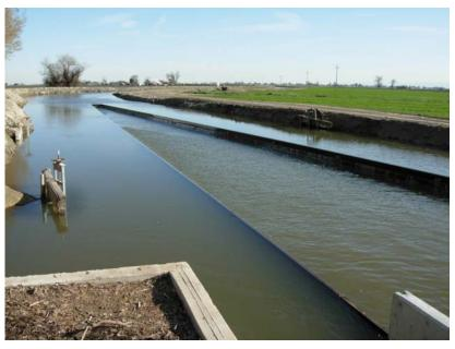
Figure 4. Very long, but simple, long crested weir at San Luis Canal Company. California has many hundreds of these structures.
