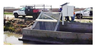
Figure 11. Automatic screen upstream of a turnout in Merced ID. Note the wall that helps prevent sand from entering the turnout.
