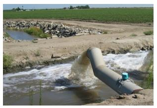
Figure 6. An elbow installed downstream of a propeller meter. In this case, the elbow is much higher than it needs to be. It only needs to be high enough to make the pipe completely full.
