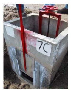
Figure 28. Alta ID rectangular orifice gate (front) provides flow measurement, while sluice gate (rear) provides flow control
