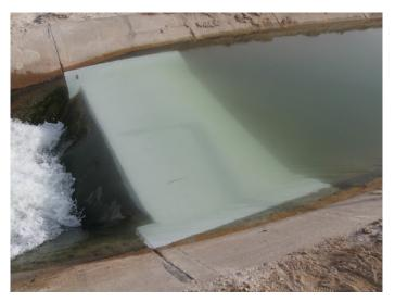
Figure 40. A flume with an ePaint<sup>™</sup> coating to minimize algae growth
