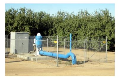
Figure 5. A loop in a pipe is installed to keep the upstream pipe section full. A continuous acting air vent is needed at the top of the loop.
