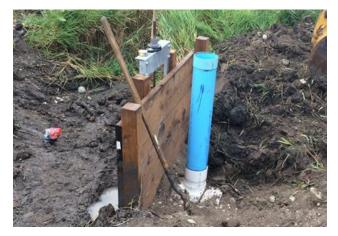
Figure 19. Stilling well installed on metergate with proper diameter, position, and height but not precast.
