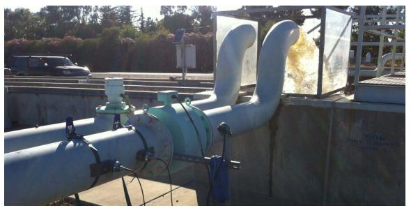
Figure 4. Water Specialties Magnetic Flow Meter at CSUC ATRC
