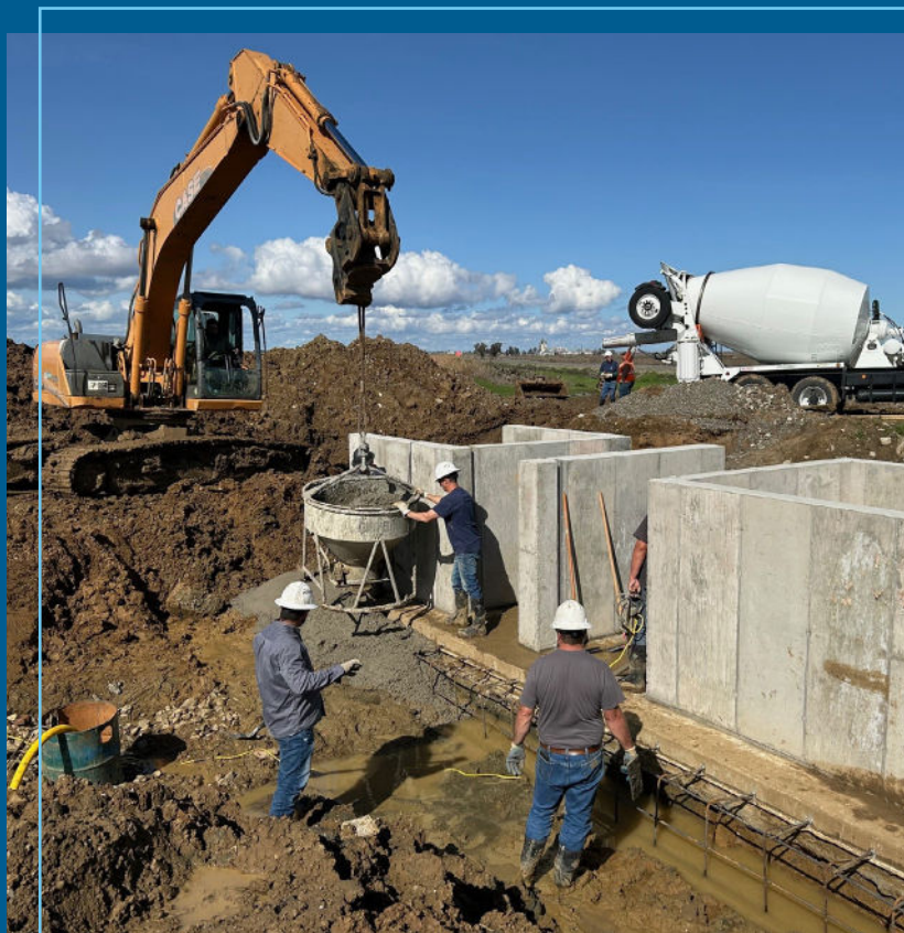
Pouring concrete floor and curtainwall on new check structures.
